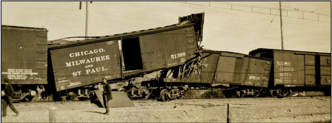
This extreme image shows why railroads spent so much time and energy figuring out how to strengthen the ends of their house cars. In this circa 1920 view, a 1916-built car to the left with steel I-beam crash posts, and a 1916-built, all-steel boxcar to the right held up fine. But the two all-wood cars between them are now kindling. Author's collection.
