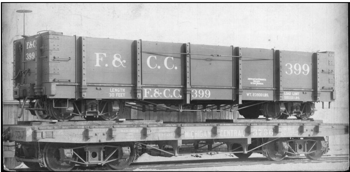
An interesting footnote to the idea of strengthening a freight car with trussrods were the few gondolas built with trussrods on their sides, in an attempt to keep them from excessively bowing outward during harsh treatment at mines. Never very popular, by 1900 the idea had been dropped in favor of all-steel gondolas. Both photos J.W. Barriger photo, St. Louis Mercantile Library collection.
