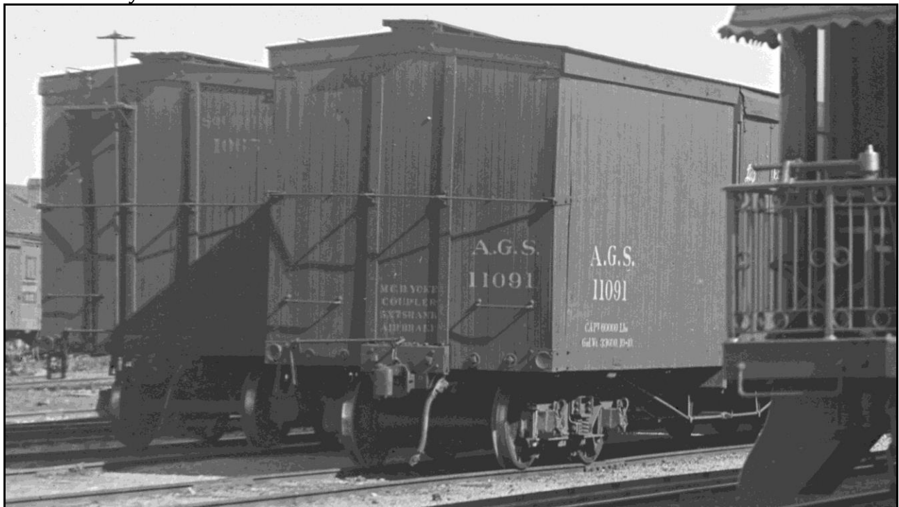
AGS 11091 is seen in Memphis, circa 1920. It's readily apparent that one of the big problems with having trussrods tied to corner braces is that when they took a hit, the entire end failed! J.W. Barriger photo, St. Louis Mercantile Library collection.
